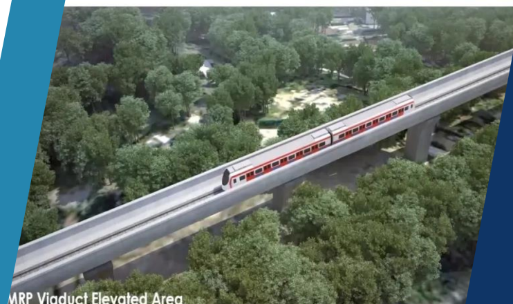
MRP Viaduct Elevated Area
