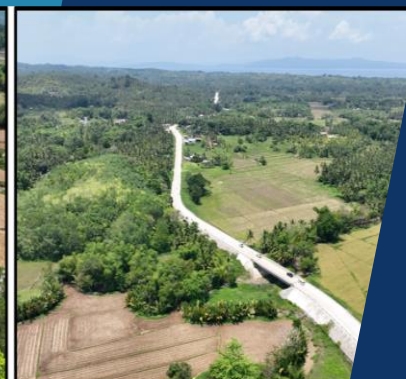
PR06: Completed PCCP Road
