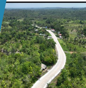
PR06: Completed PCCP Road
