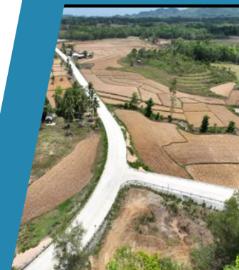
PR07: Completed PCCP Road
