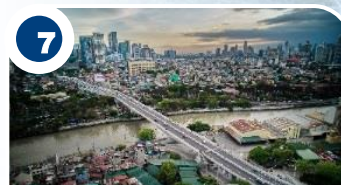
BGC-Ortigas Center Link Road Project
