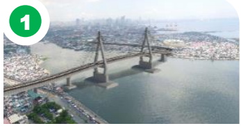
North-South Harbor Bridge *
