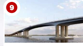
9 Cebu-Mactan Bridge (4th Bridge) and Coastal Road Construction Project (8.68 km)
