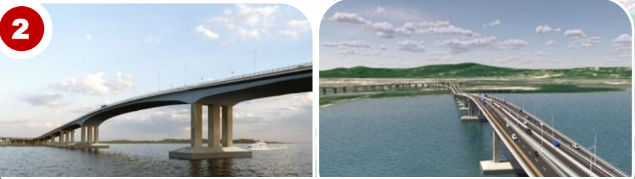
2 Cebu-Mactan Bridge (4 th Bridge) and Coastal Road Construction Project (8.68 km.)
