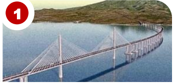
1 Bataan-Cavite Interlink Bridge (32.15 km)
