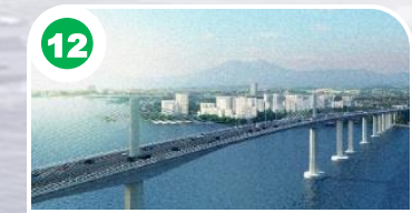
12 Samal Island-Davao City Connector Bridge 4.01 km)
