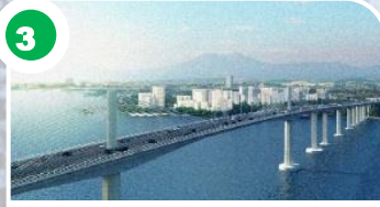
Samal Island-Davao City Connector Bridge (4.01 km)
