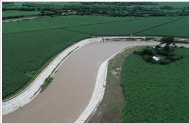
Slope Protection along Binalbagan River, Hinigaran, Negros Occidental
