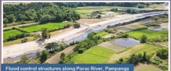
Flood control structures along Porac River, Pampanga
