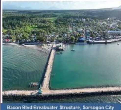
Bacon Blvd Breakwater Structure, Sorsogon City
