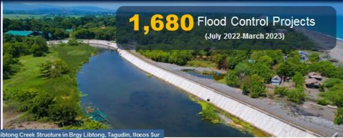
Libtong Creek Structure in Brgy Libtong, Tagudin, Ilocos Sur
