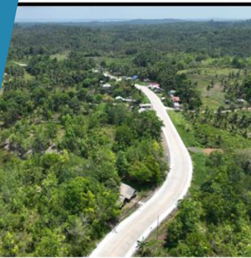
PR06: Completed PCCP Road
