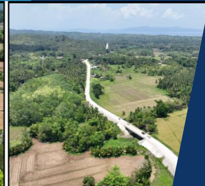
PR06: Completed PCCP Road
