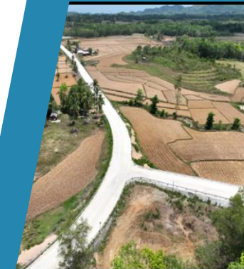
PR07: Completed PCCP Road
