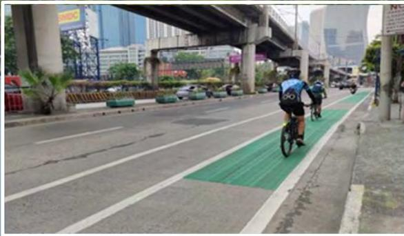
Completed 100% of the 497 km bike lane networks in METRO MANILA, METRO CEBU, AND METRO DAVAO with pavement markings, bollards, curbs, and solar studs.
