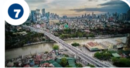
BGC-Ortigas Center Link Road Project
