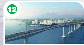
12 Samal Island-Davao City Connector Bridge 4.01 km
