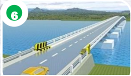
6 Malassa-Lupa Pula Bridge, Tawi-Tawi (0.68 km)
