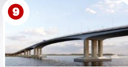
9 Cebu-Mactan Bridge (4th Bridge) and Coastal Road Construction Project (8.68 km)
