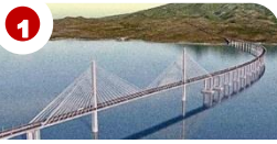
1 Bataan-Cavite Interlink Bridge (32.15 km)
