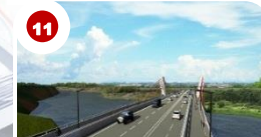
Kabayani St. - Matandang Balara Bridge
