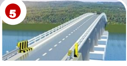
5 Tongsinah-Paniongan Bridge, Tawi-Tawi (0.57 km)
