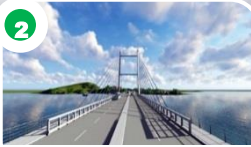
2 Panglao-Tagbilaran City Offshore Bridge Connector (2.71 km)
