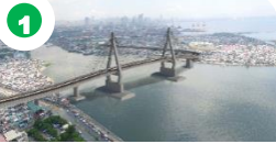
North-South Harbor Bridge *
