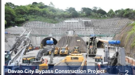
Davao City Bypass Construction Project
