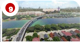
Marcos Highway - St. Mary Ave. Bridge
