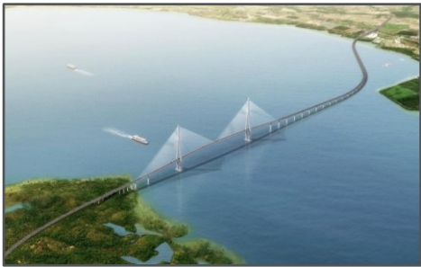
Panay-Guimaras-Negros Inter-Island Link Bridge – PHP187.5bn (US$3.3bn)
