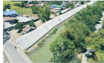
This involves the construction and maintenance of drainage/slope protection works for national roads and bridges, major components of urban drainage systems, including drainage mains, outfalls, pumping stations, control gates, and dredging and improvement of major drainage channels.
